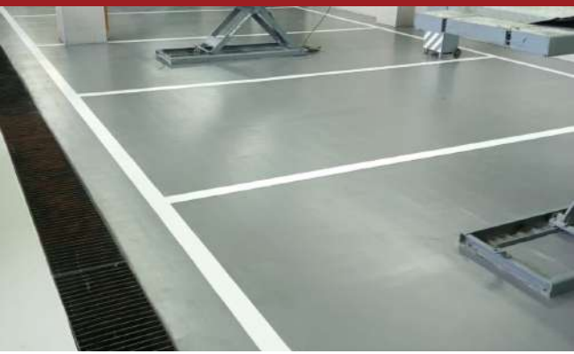
Performance Flooring - BMW TB Simatupang
