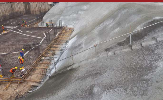
Shotcrete - Kt&g Indonesia
