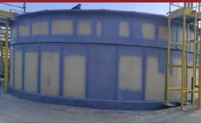
Fiber Strengthening - Amman Mineral Nusa Tenggara
