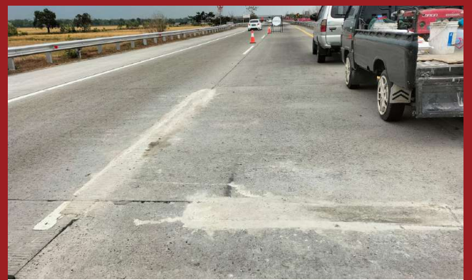
Concrete Repair - Tol Mojokerto Jombang
