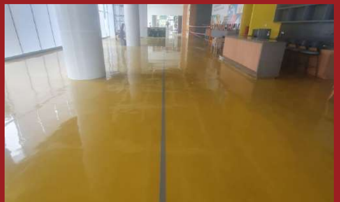
Flooring Coating - Gedung Adira Finance
