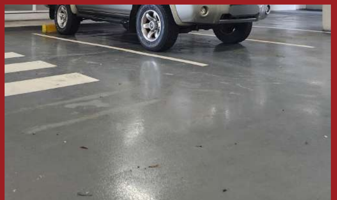
Waterproofing - Tunjungan Plaza 6 Carpark Area
